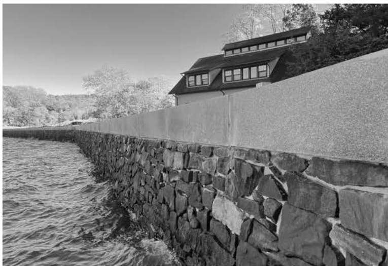
CSHL's new seawall is two feet taller than its predecessor. It is constructed from the same kind of heavy-duty concrete used in skyscrapers and features a facade comprised of stones from the original seawall built in 1850.
