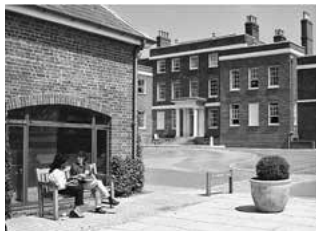
Conference Center and Hall, side view
