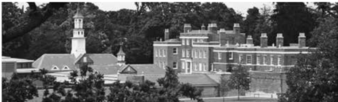
Wellcome Trust Conference Center, Main Conference Center and Hinxton Hall
