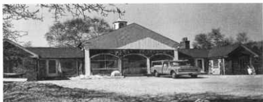
The garage during renovations.
