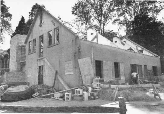
Power House renovations
