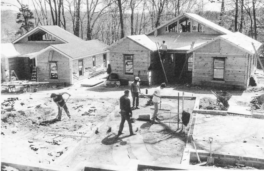
Guest cabins under construction
