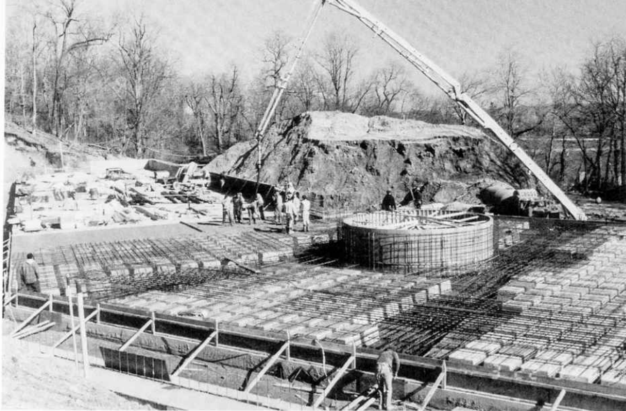
Neuroscience Center under Construction
