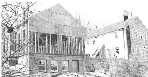
Delbrück Laboratory under construction
