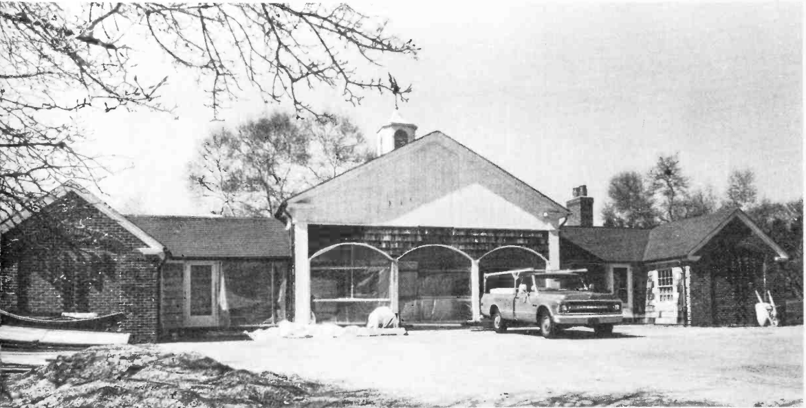
Banbury Conference Center under construction
