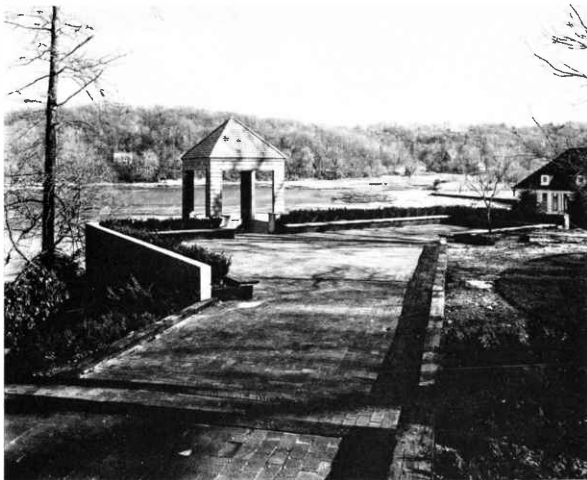
The gazebo atop the new waste-water treatment plant. (Photo by Norman McGrath)
