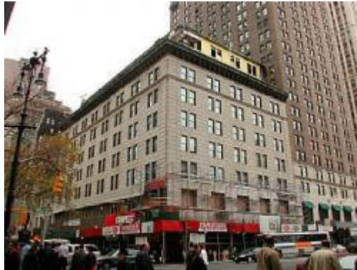
217 Broadway in Manhattan was originally built by John Jacob Astor as a fashionable hotel. Photographer Matthew Brady lived there and philosopher William James was born there. Abraham Lincoln slept there during his campaign for the Presidency. To the immediate left of 217 Broadway is St. Paul's Chapel. About two buildings to the right of 217 Broadway is the Woolworth Building at 233 Broadway, one of the first skyscrapers of New York City.
