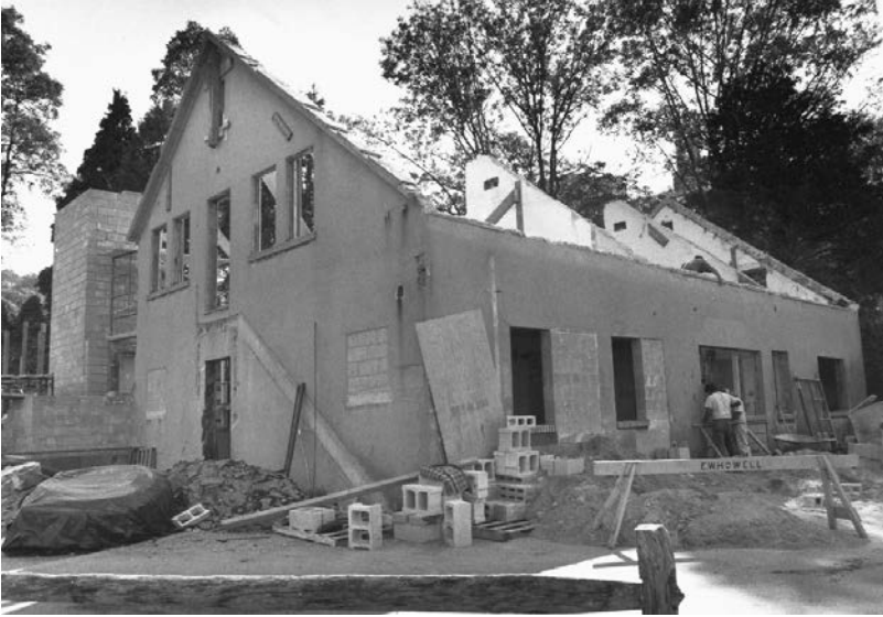
Power House renovations
